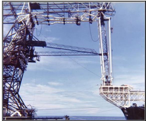
Figure 1 Shell Brunei LNG Loading Facility
