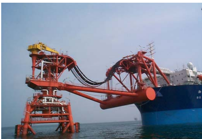
Figure 1: Tower Yoke Mooring System
