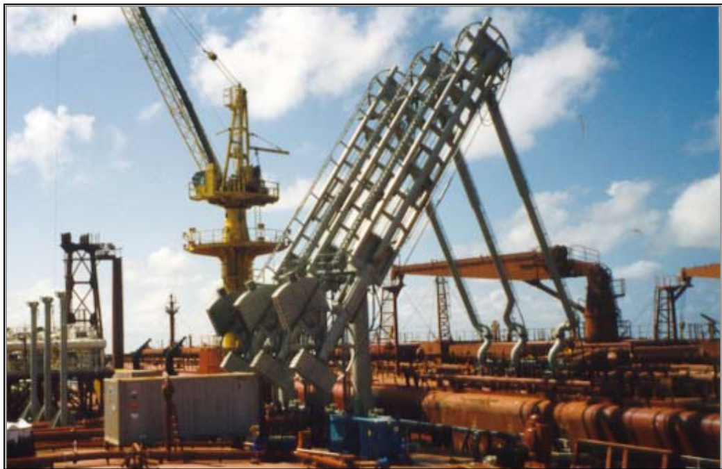
Figure 3: Offshore Ship-to-Ship Transfer Loading Arms
