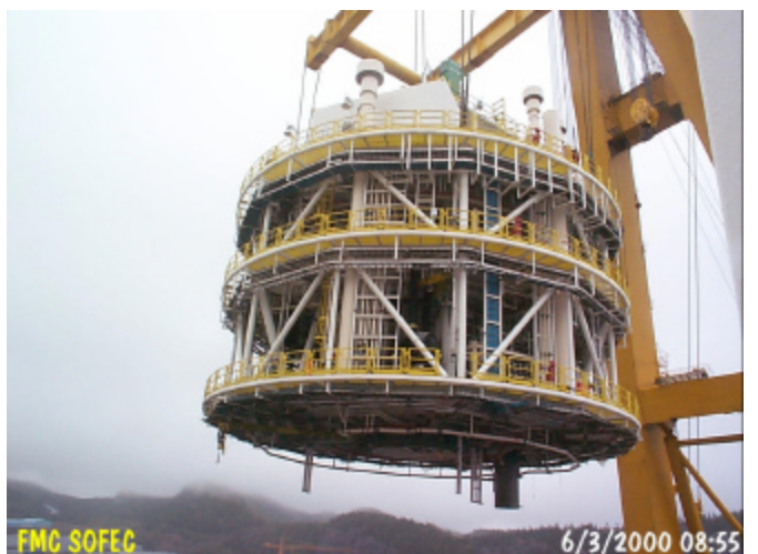
Figure 8 – The Upper Turret Structure being Installed on the FPSO
