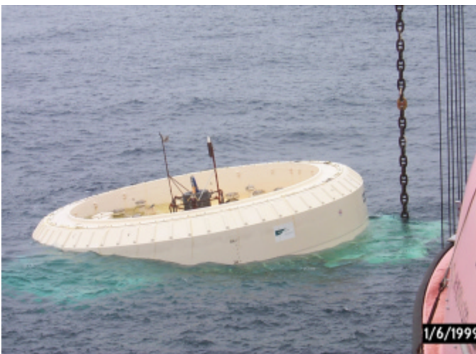
Figure 7 – Installation of the Spider Buoy
