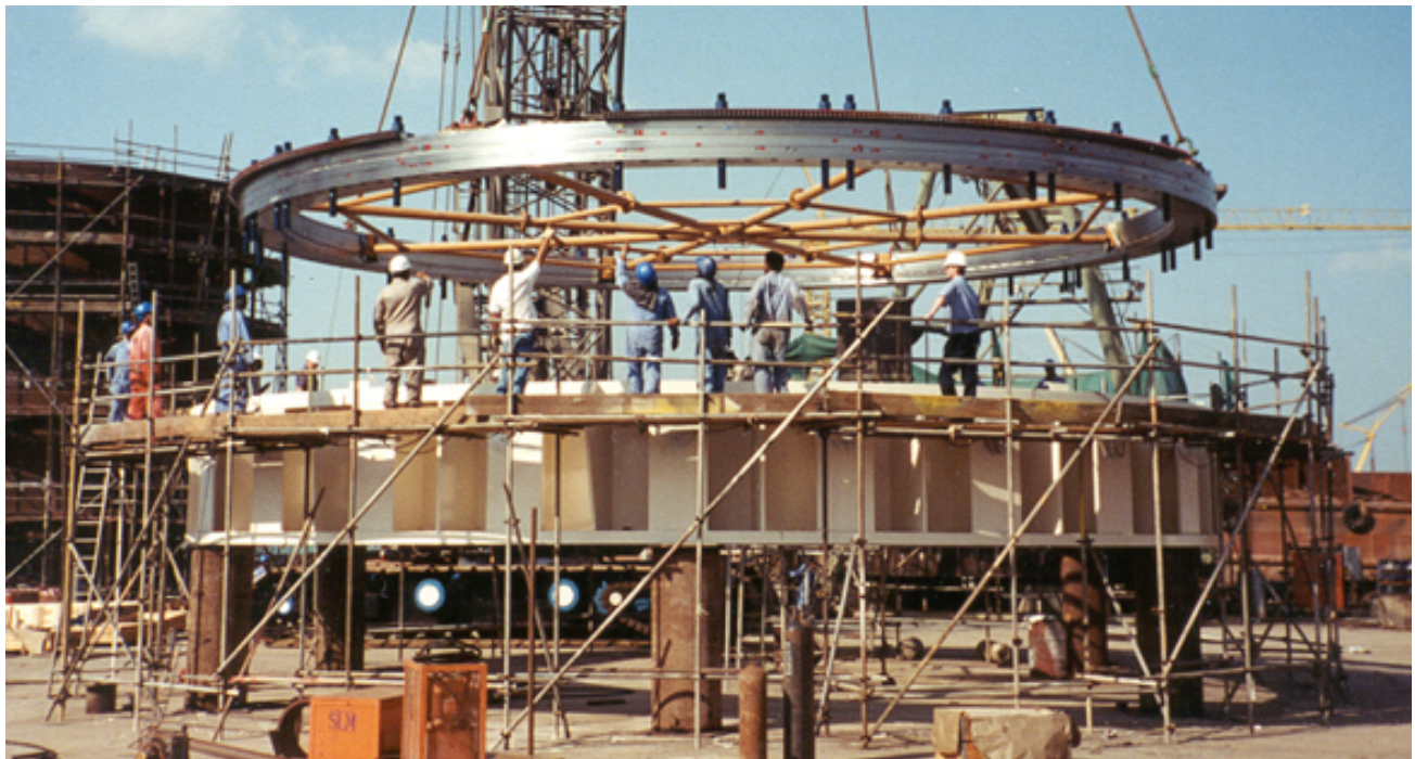
Figure 4 – Installation of the Main Bearing
