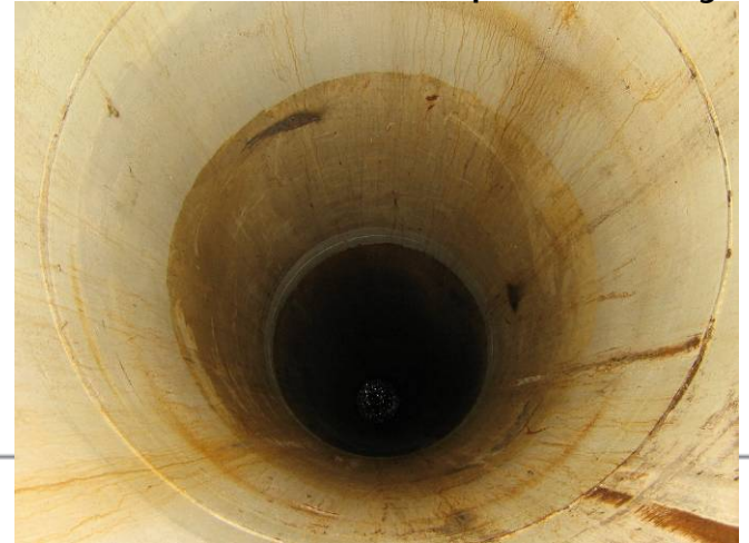
Riser Lowered to Spider Buoy
