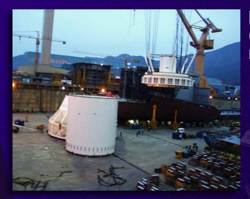
Lower turret module (TS1) inserted in ships moon pool keel block
