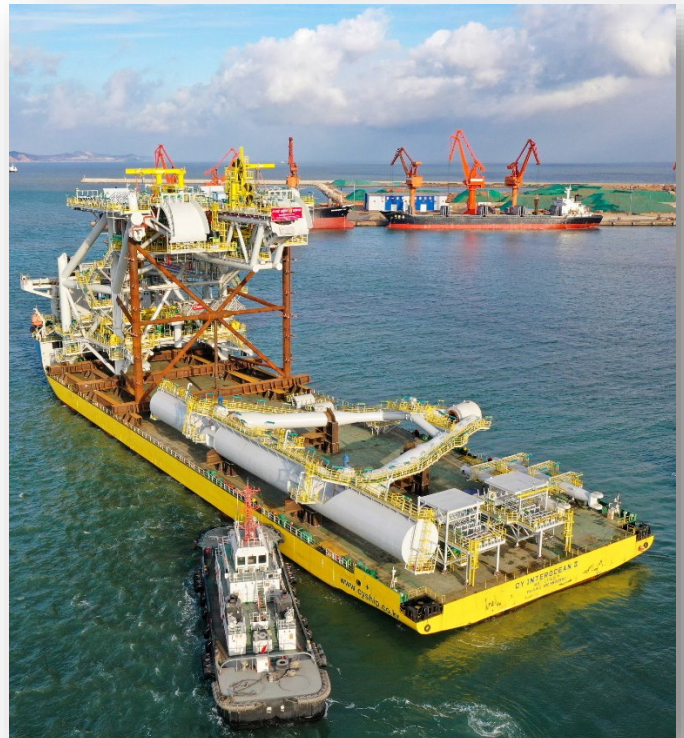
MSS & Yoke structure on its way to integration yard
